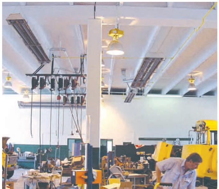
A highly radiant efficient Space-Ray infrared heating system can normally save a building owner 30% to 50% in annual fuel costs compared to forced air heating systems.
